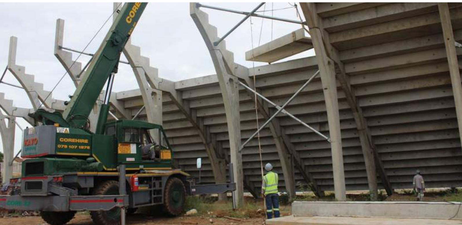
The system comprises pre-cast concrete columns, raker beams, seating benches and side panels that are installed by our team once earthworks and site terracing for the stadium is completed by the main contractor. After casting the concrete bases and installing the connection bolts, the columns are fixed in position and aligned, ahead of the placement of the raking columns and seating benches.
