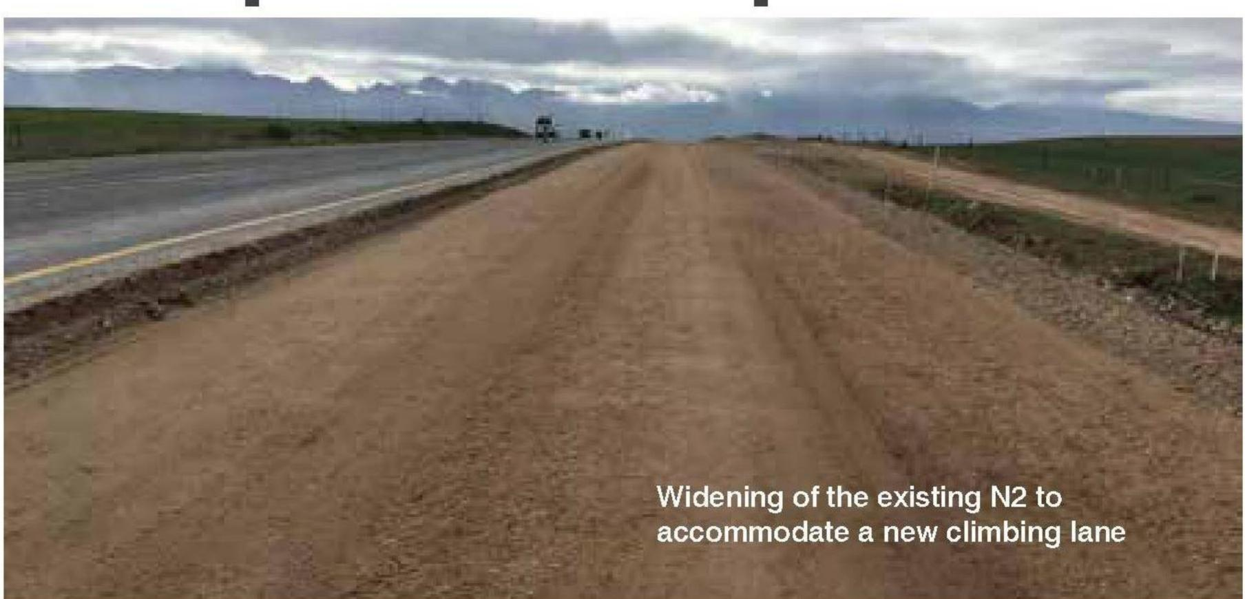
G Afrika is overseeing the upgrade of a 48 km section of the N2 highway between Caledon and Riviersonderend in the Western Cape, with the works being carried out by main contractor Group Five. The main scope entails the widening of the road, which was originally built between 1978 and 1983, as well as upgrading its intersections to accommodate increased traffic volumes.
