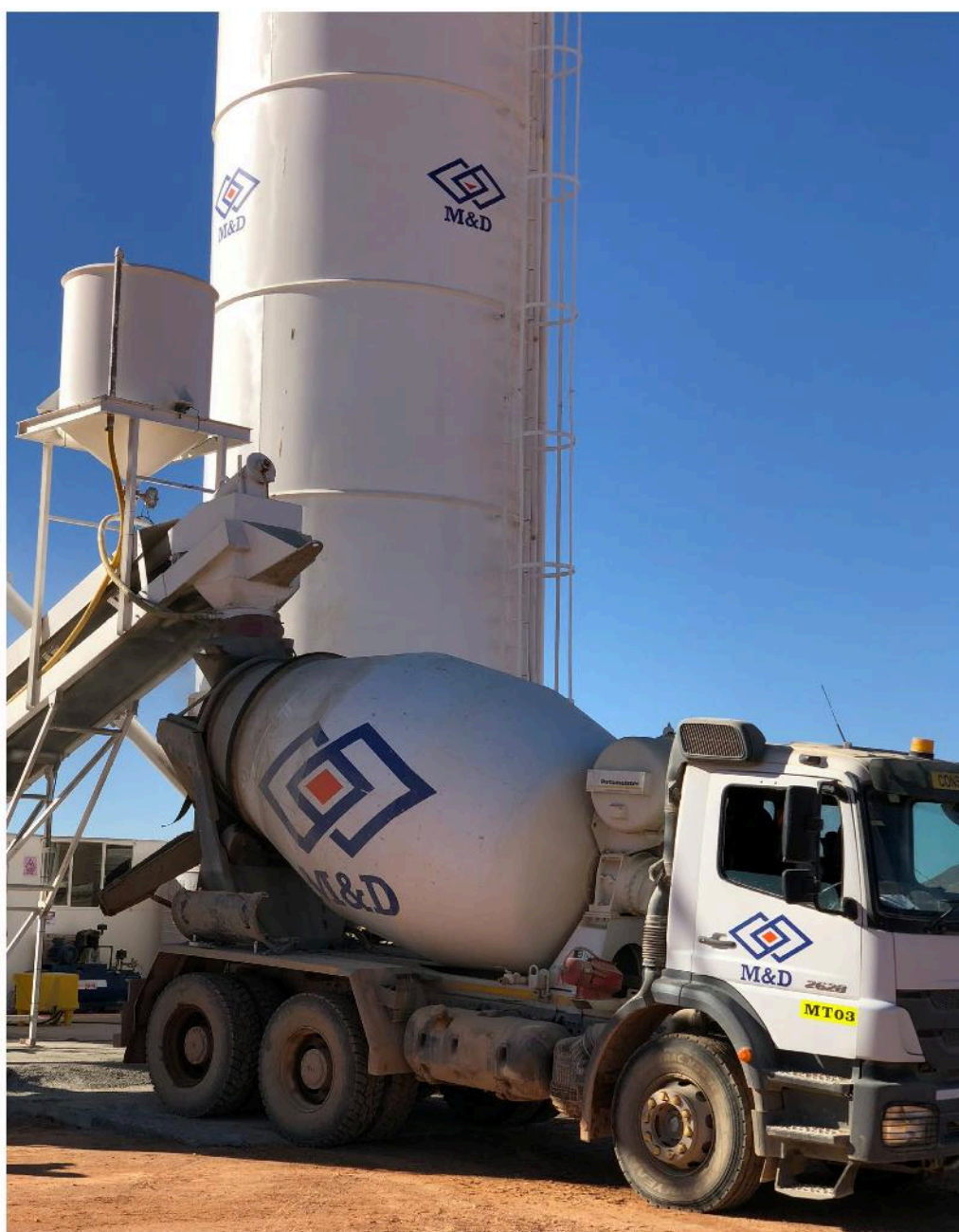
Concrete for the concrete roadways is being produced from M&D Construction Group's batch plant on site and transported to the various construction faces by the company's own three-mixer trucks
