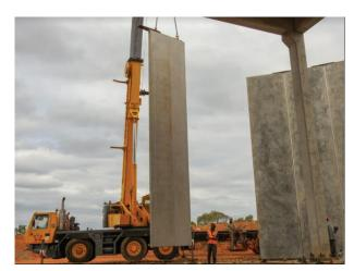
Corestruc is able to construct the walls and roof in as little as three months on site, while the manufacture of the structure takes place at the factory during the earthworks and construction of the foundations.
